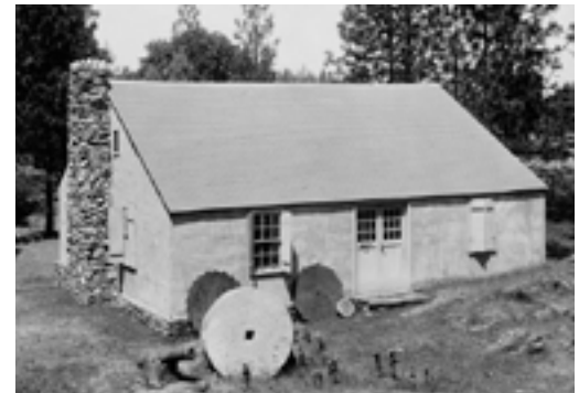
Historic American Buildings Survey Wells Fargo Bank Historical Museum, S.F. Original: June 1926 Re-photo: August 1940 - James W. Marshall Blacksmith Shop, Kelsey, El Dorado County, CA
